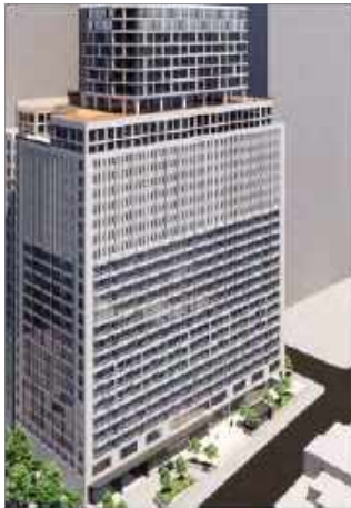
Existing office building
